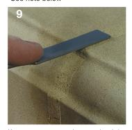
If necessary trowel over the joint once more to ensure a flush finish.
