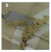
Scoop the mix into the joint, pressing with a trowel to ensure an even fill.
