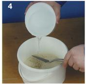
Carefully add small quantities of water to the Humber Cast Stone pointing mix, mixing thoroughly to ensure the water is fully dispersed.
