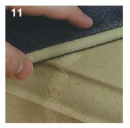
Any mix residue may be rubbed away with fine abrasive paper 2-3 days after completion.
