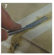
Smooth the pointing mix to the profile of the stone, removing any excess pointing mix.
