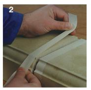
Apply masking tape to both sides of the joint, keeping the tape approximately 1mm ( $^{1}/_{16}$ ") from the edge of the joint.
