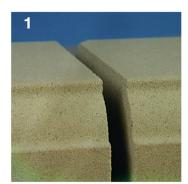
Before pointing ensure each 6mm (¼") joint is free from loose particles. Avoid pointing in extreme conditions, particularly wet and
