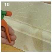
Apply a fine and even mist of water to the joint to prevent drying out.
