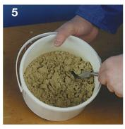
The Humber Cast Stone pointing mix is ready when it has the consistency of damp sand. \*See note below
